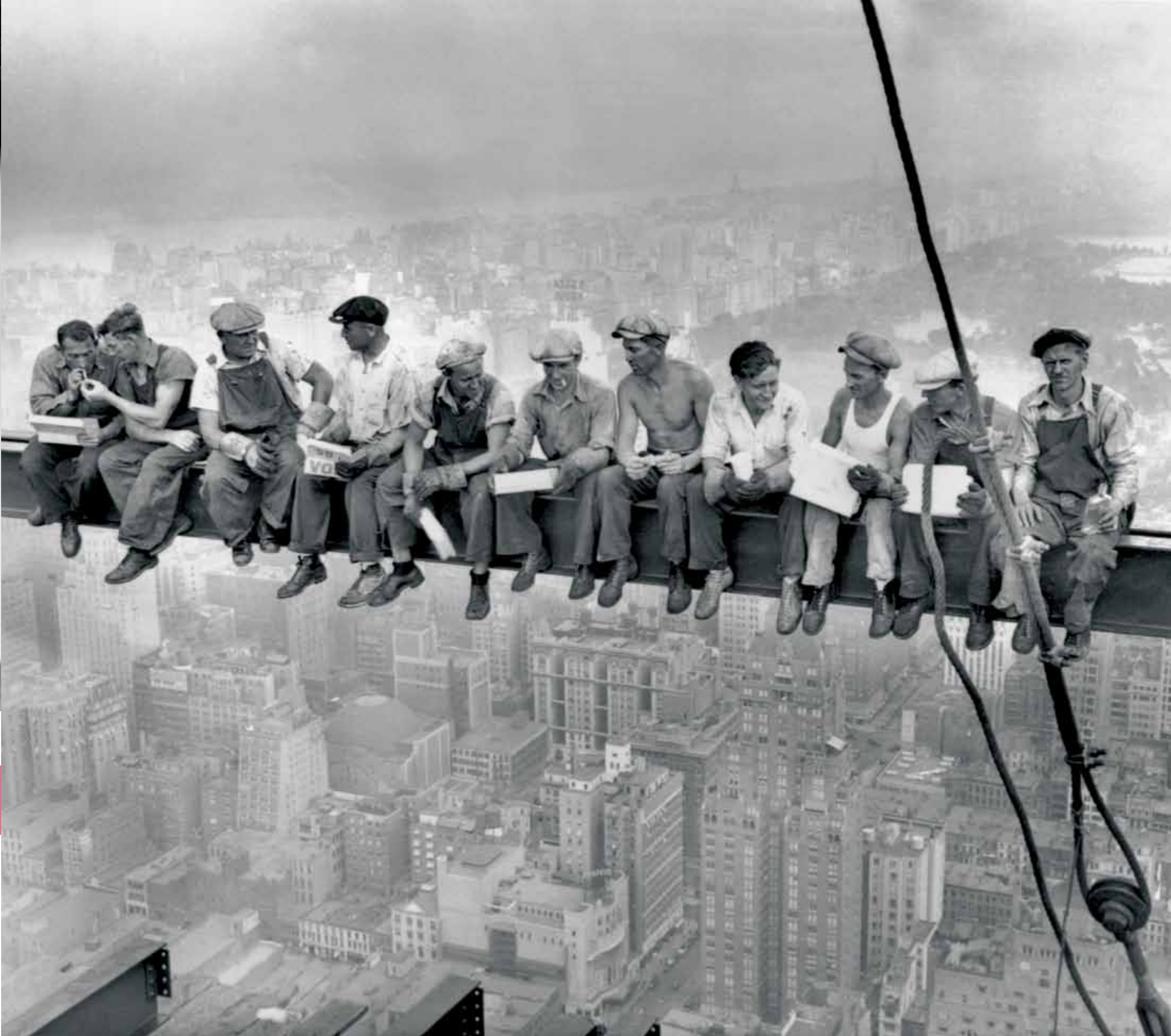
Construction Workers Lunching on a Crossbeam, 1932. Photograph by Charles C. Ebbets. © Bettman/Corbis
